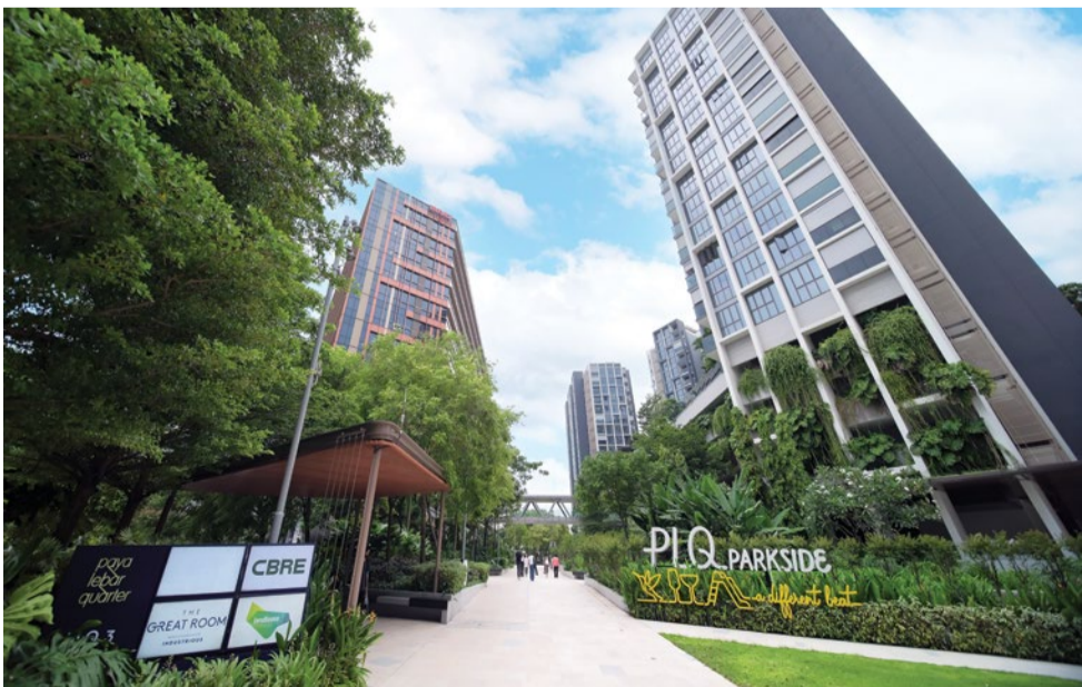
Lendlease has embedded placemaking at Paya Lebar Quarter (pictured), participating in URA’s Business Improvement District pilot programme to activate public spaces and shape precinct identity
